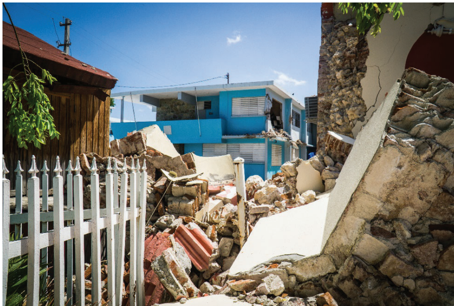
Figure 2: Damage from 6.4 earthquake on January 7, 2020 in Guayanilla
